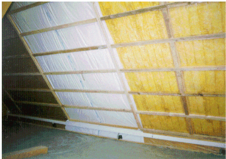
Figure 11 The tested roof covered with metal sheets. Top: Basic design of the test sections. Bottom: Photographical view of the interior
