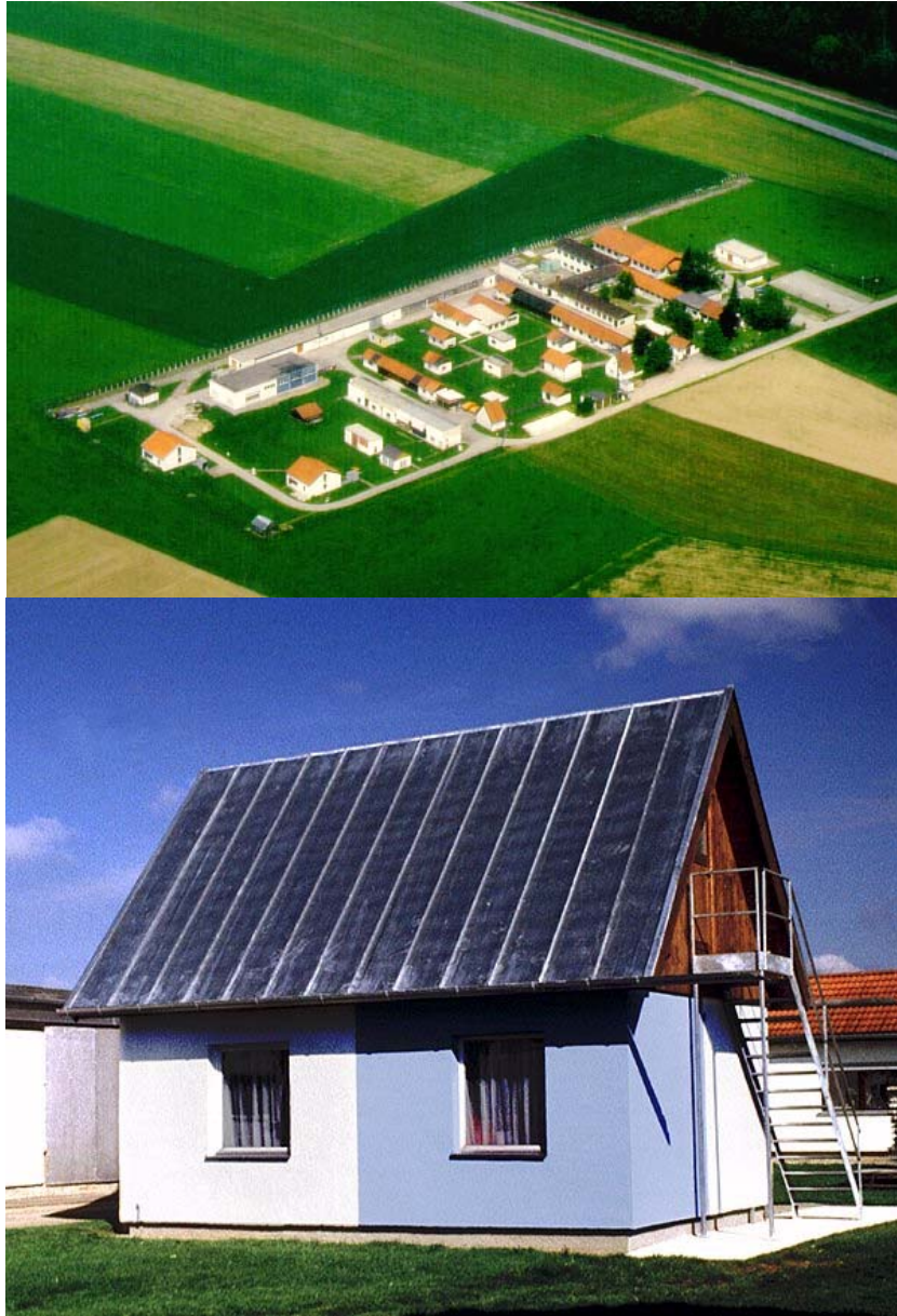
Figure 1 Field testing area in Holzkirchen, Germany Top: Photographic view of the whole area Bottom: Photographic view of the building with roof made of metal sheets
