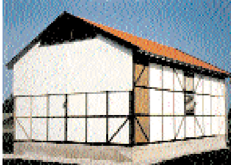
Timber-framed building on the outdoor area at IBP.
