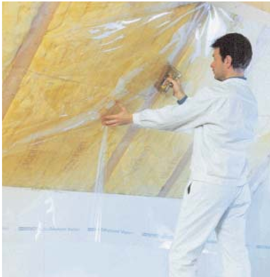
The moisture barrier is quickly and easily applied.
